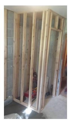
The above photo again shows the lack of a header and the fresh concrete that has been applied over the excavated plumbing.
