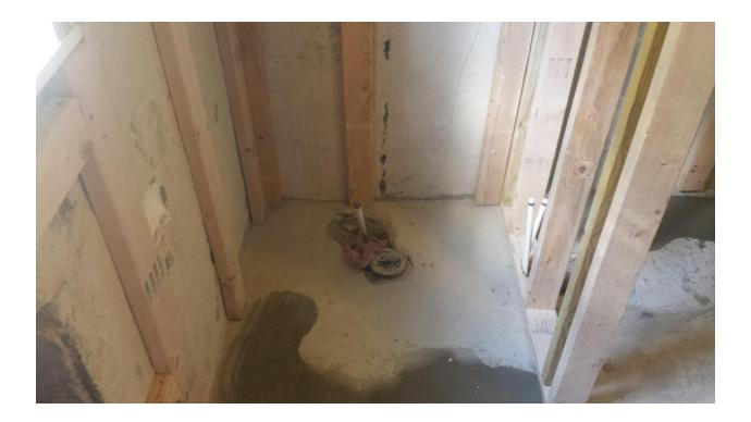
The above photo shows the area where the toilet is to be located. The contractor has placed the water supply line and used the old flange and drain for the toilet. The 2x4's placed against the wall flat in this manner used as furring strips reduce the backset for toilet placement which will cause problems when the toilet is to be set. It will not allow enough space to set the toilet once the wall is finished.
