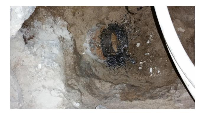
The above photo shows the sever line below the toilet as Bruhl Construction attempts to remove the original steel sewer line after cutting off the bad portion... This piece had to be drilled and chipped away in small pieces to keep from damaging the service pipe so it could be connected to and used for the toilet and shower. The above work took several days alone to complete and should have been done by the first contractor when it was discovered.
