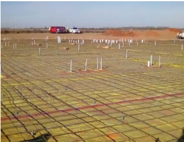
High school Area C slab pre-pour
