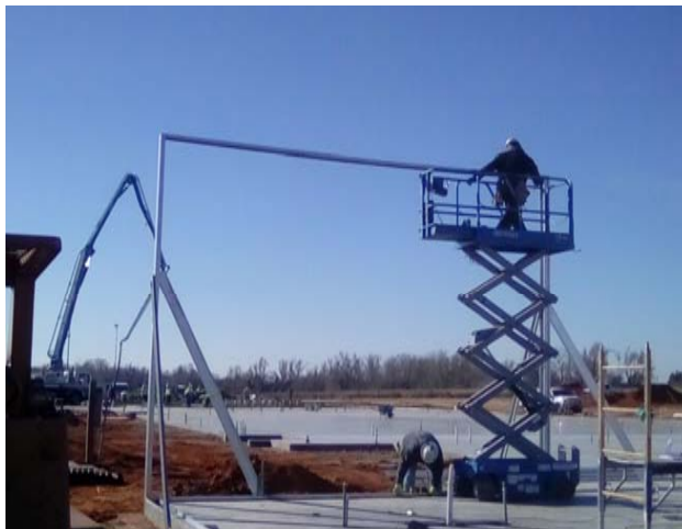
High school Area A structural wall framing begins
