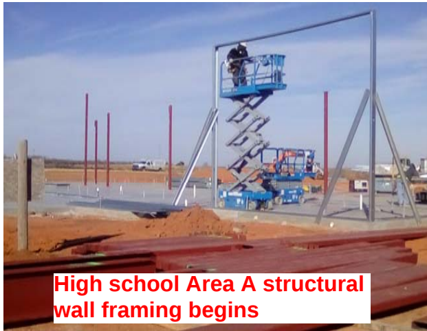
High school Area A steel erection has begun
