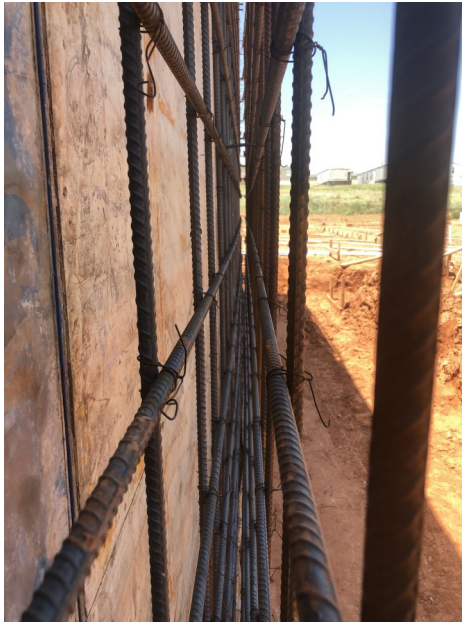
Shelter Reinforcement Doorway Embeds West Elementary
