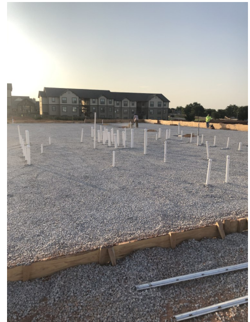
Floor with gravel subbase and vapor barrier
