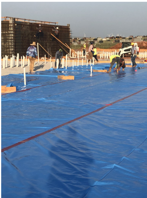
Floor with gravel subbase and vapor barrier
