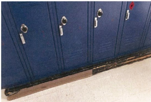
Figure 4: Locker base and baseboard
