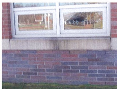
Figure 7: Precast sill
