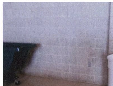
Figure 4: Cafetorium CMU wall
