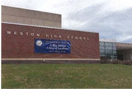
Figure 1: View of High School main entrance
