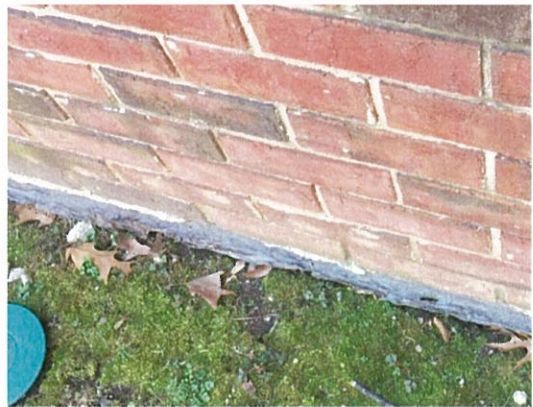
Figure 13: Through wall flashing condition at North House
