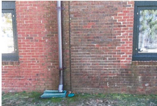
Figure 12: North House masonry conditions
