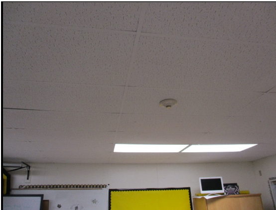
Fire alarm system-smoke detector in classroom
