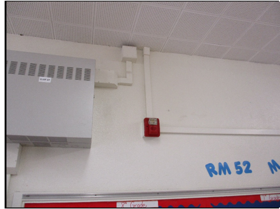
Fire alarm system, strobe and horn
