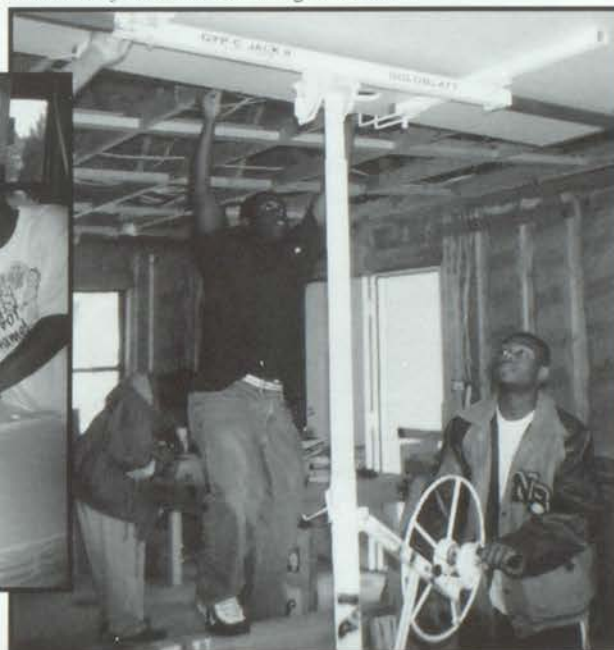
Horatio McChester helps Ryan Wade hang sheetrock.
