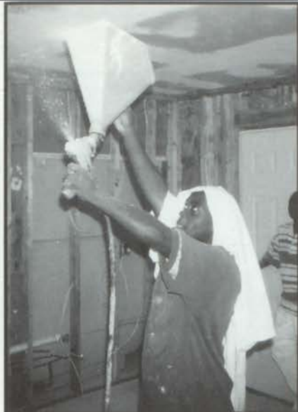
Ryan Wade blows the ceiling texture on the ceiling.
