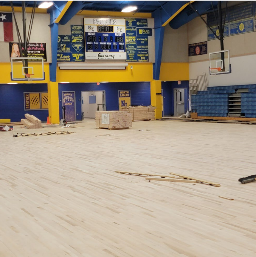
NLHS gym floor in progress
