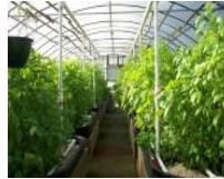
Nursery, Sod, Greenhouse
