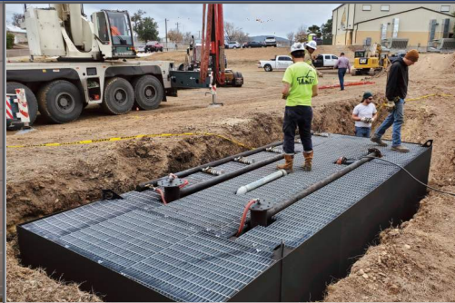
New Sewer Plant 01.15.2020
