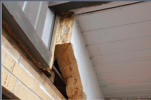
Exterior Beam Repair 01.15.2020
