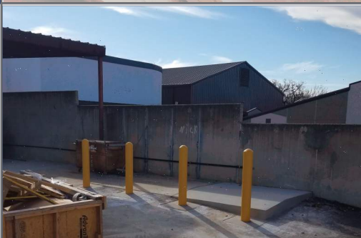
Propane Tank Concrete Pad 01.06.2020
