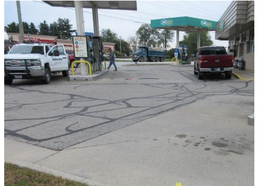
Photo 38 – Fuel dispensers at the Lassus Handy Dandy adjacent to the southeast of the site, looking to the west
