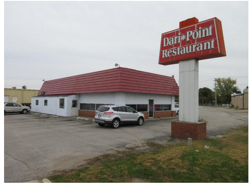
Photo 14 – View of the restaurant building on the south-central portion of the site, looking to the northeast
