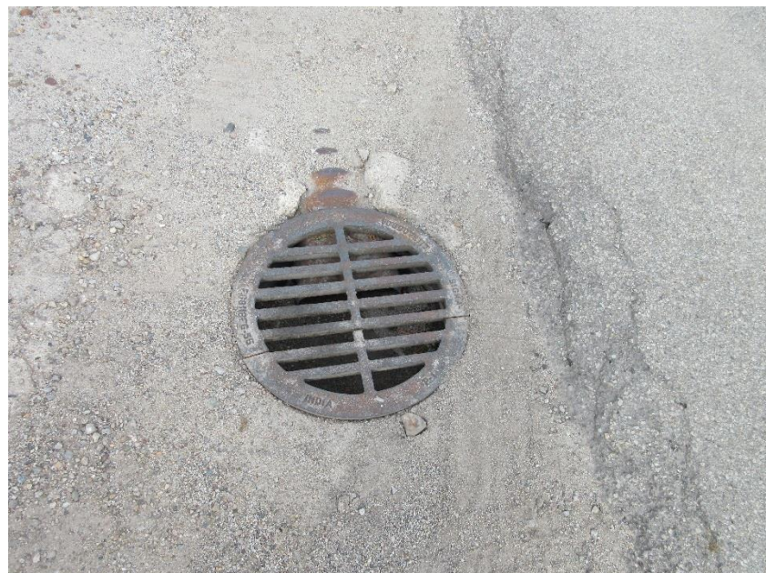
Photo 30 – Storm water drain east of the church building on the southwest portion of the site
