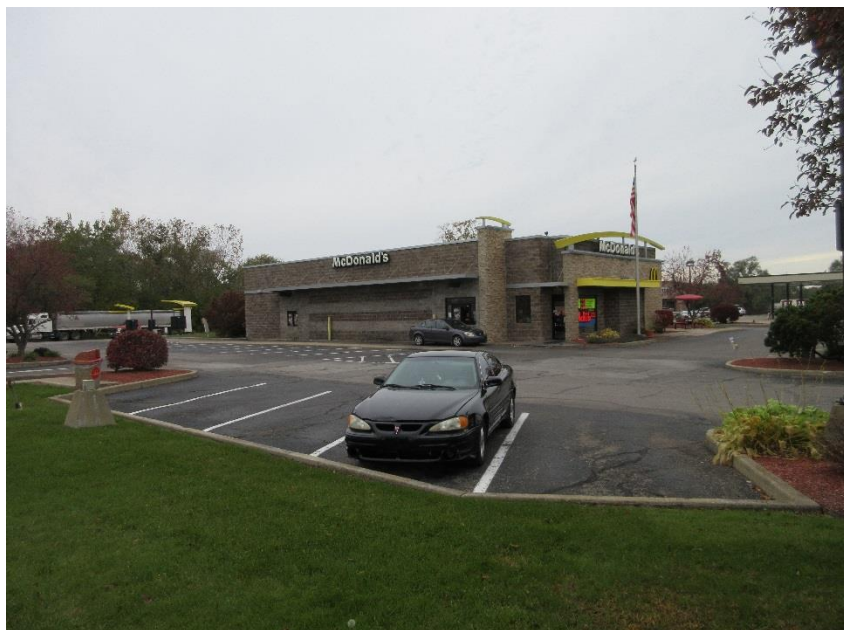
Photo 31 – View of the McDonald's restaurant adjacent to the north of the east portion of the site, looking to the northwest
