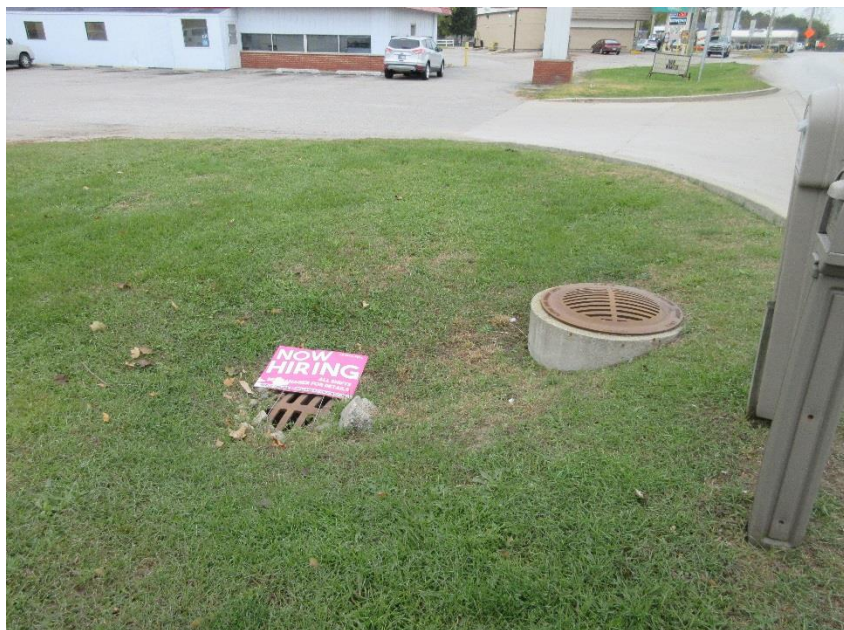
Photo 29 – Typical storm water drains along the site perimeter
