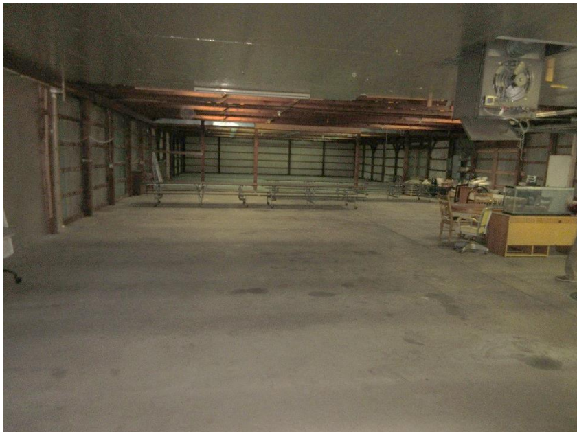
Photo 23 – Meeting hall and storage areas for the church in the central and north portions of the southwest site building
