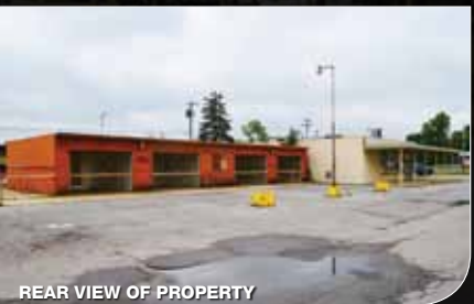
REAR VIEW OF PROPERTY
