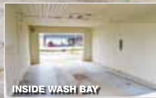
INSIDE WASH BAY
