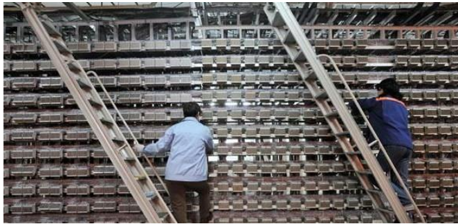
Figure 4-1 Subscriber Copper Lines at the Central Office
