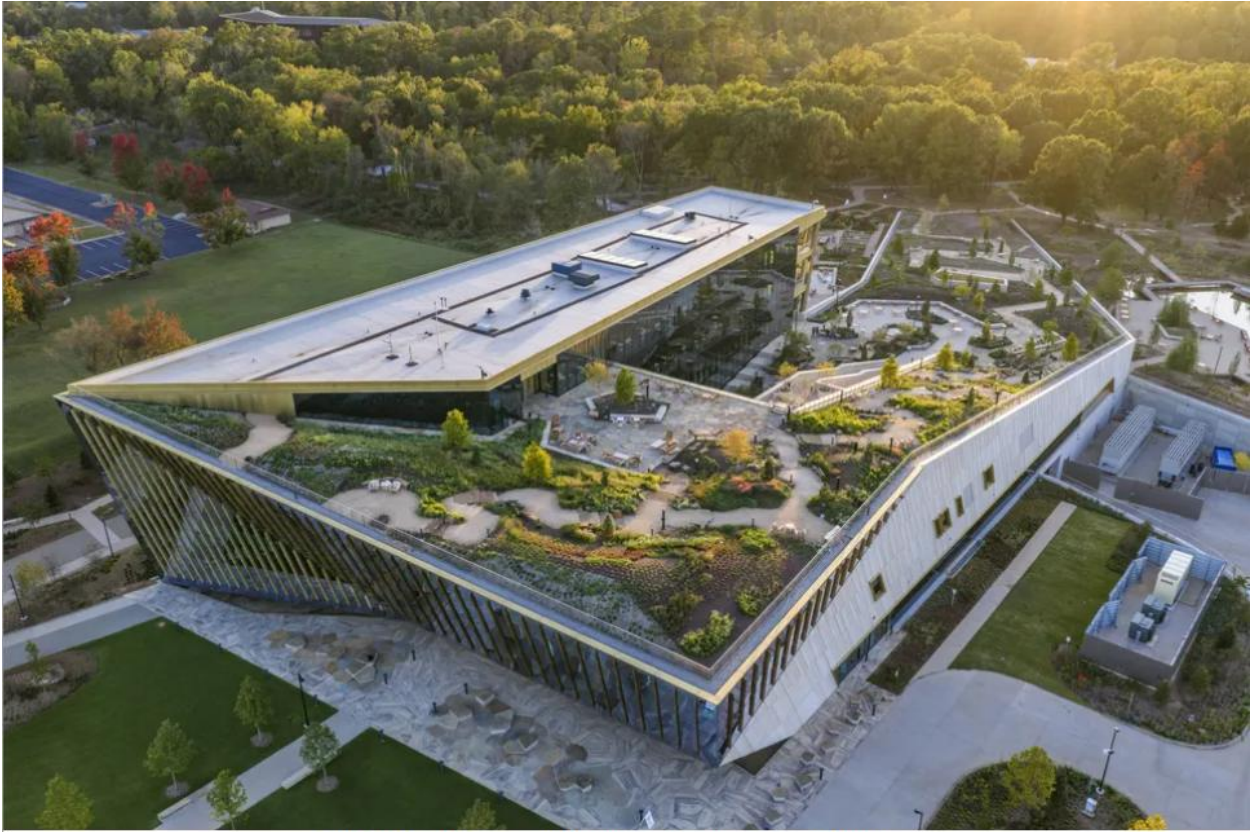
The School of Medicine showcases a green roof and extensively landscaped grounds that reflect its nature-themed approach. Photographer: Timothy Hursley
