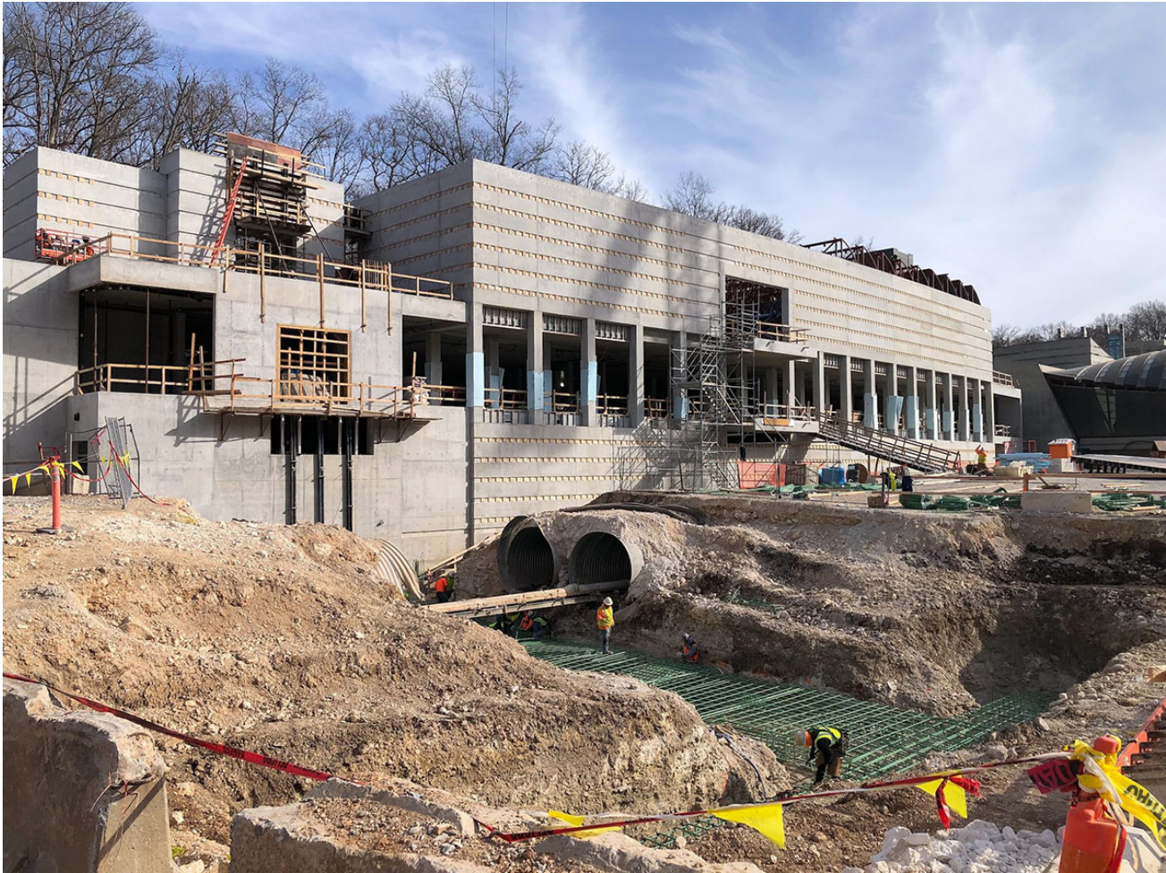
The new Learning & Engagement Hub and exhibition gallery under construction is seen in this photo from April. (Provided)
