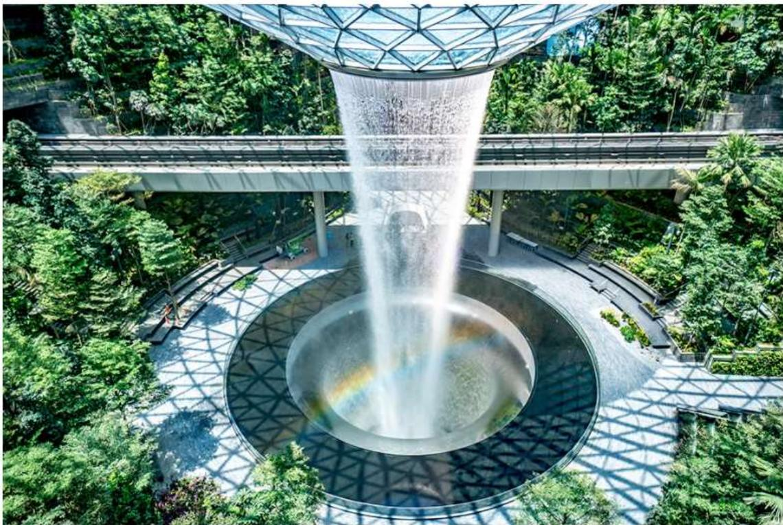
Jewel's "Rain Vortex," engineered by WET, towers at 130 feet. During Singapore's frequent storms, up to 10,000 gallons of rainwater per minute cascade through the oculus. This water is recycled throughout the building.
