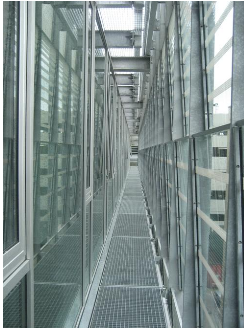
Fig 4.16- Air space between internal and external layers.
