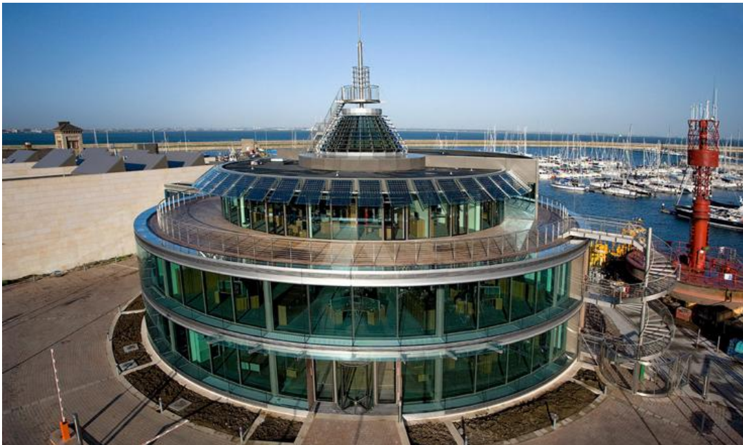
Fig 4.12- Commissioner of Irish Lights building.
