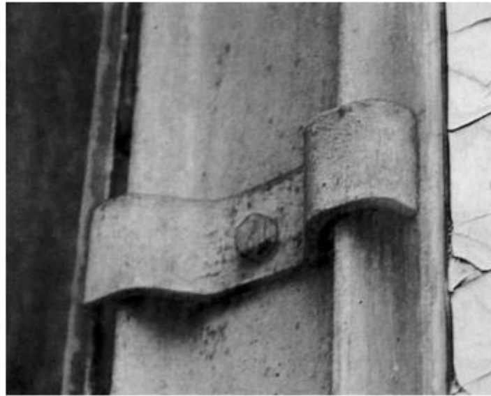
Fig 2.6- Butt straps punctually attached
