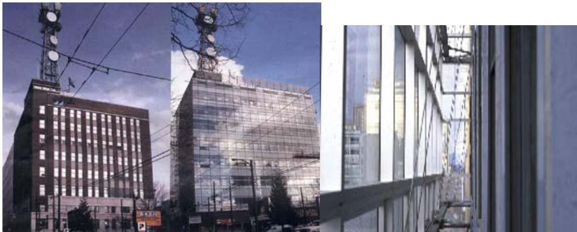
Fig 3.7/3.8- Telus William Farrell building, Vancouver.
