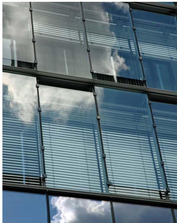
Fig 3.13- Shading devices located in air space
