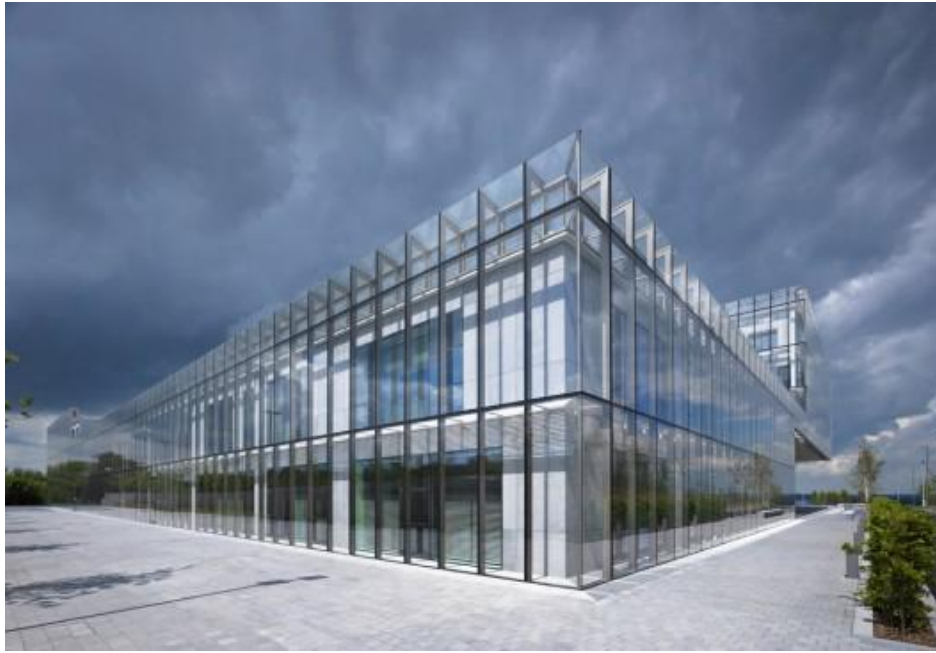
Fig 4.5- Back of Wexford County Council Headquarters.
