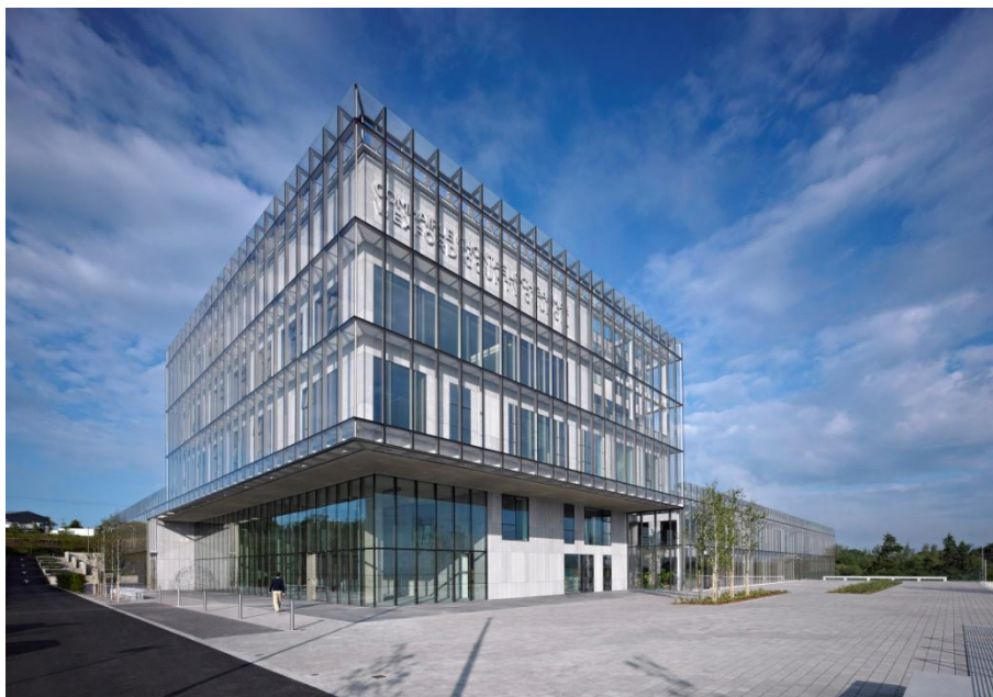
Fig 4.4- Wexford County Council Headquarters.
