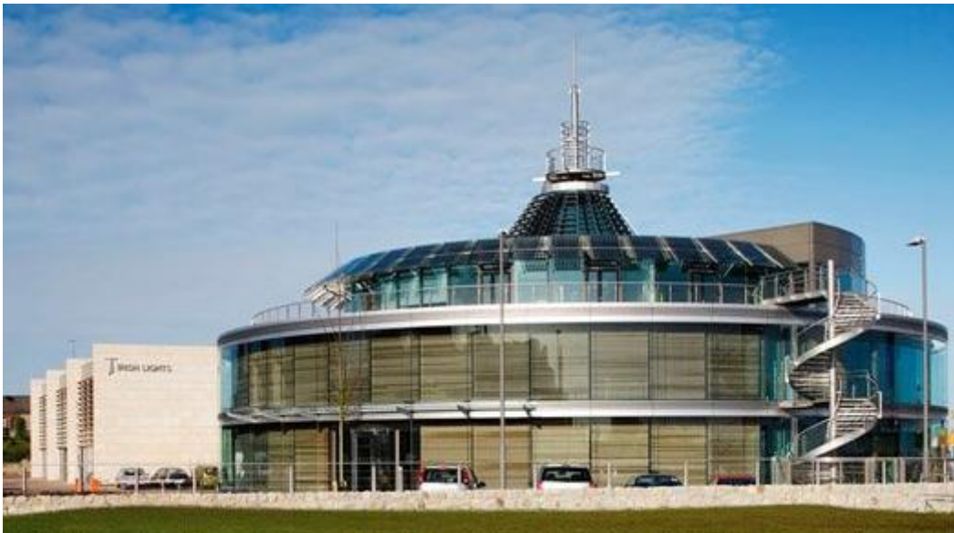
Fig 4.13- Commissioner of Irish Lights building.
