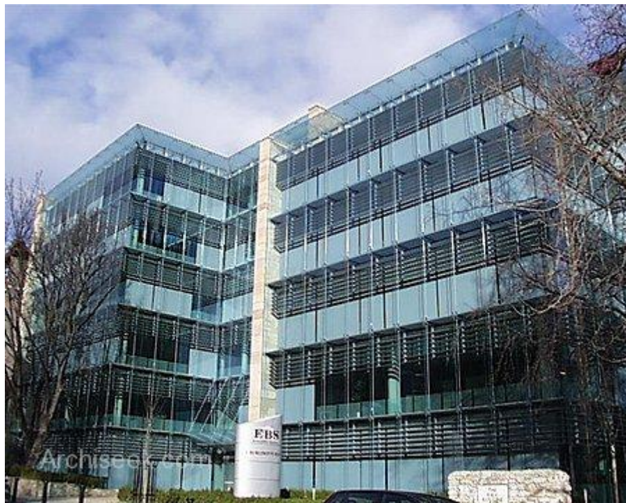
Fig 2.10- EBS building, Burlington Road, Dublin
