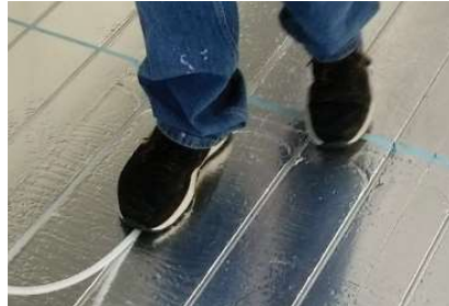
Figure 13: Press pipe into the groove
