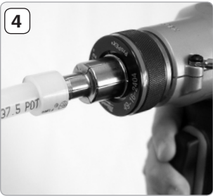
Expand the Tubing
