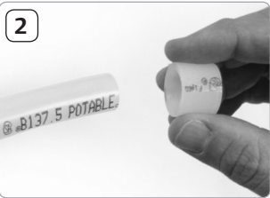
Slide ProPEX Ring onto Tubing
