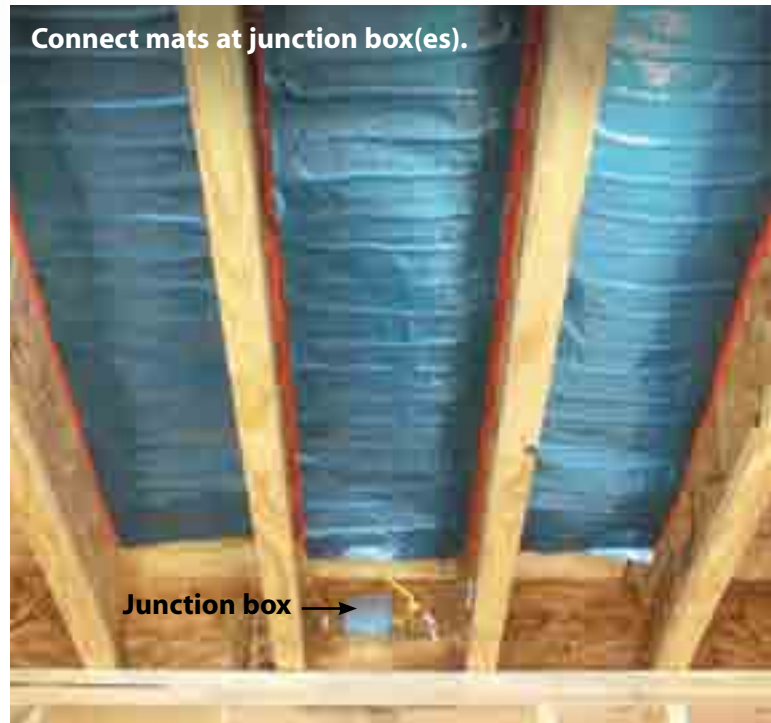
Install insulation.
