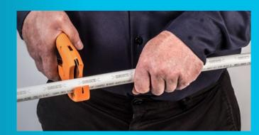
Step 1 Cut the desired length of pipe.
