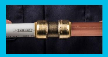
Step 4 Push the tubing into the fitting.
