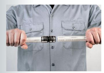
Step 3 Push the pipe into the fitting firmly.
