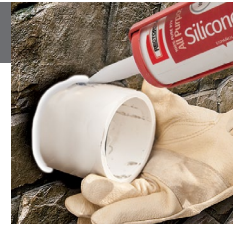
Caulk wall opening.
