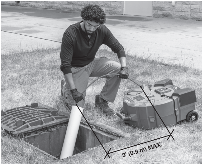
Figure 9 – Example of Extending Drain Access to within 3' (0.9 m) of Machine Cable Outlet
