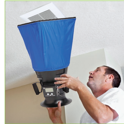
Balometer used to verify installed performance
