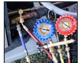
**NOTE:** You may also use a refrigerant cylinder to push sealant into system while charging if the system is low on refrigerant. Just connect EasySeal Ultimate to service port and inject refrigerant through injector into system while charging.
