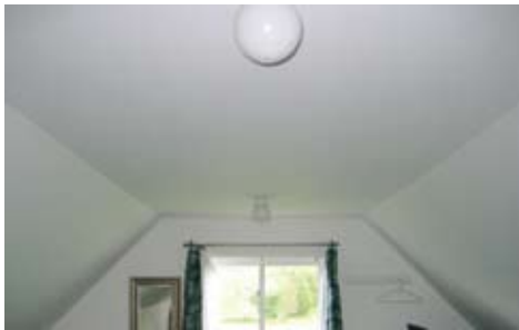
finished radiant wall
