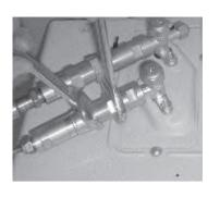
the warranty. during installation may void to use the appropriate tools copper from twisting. Failing opposing side to prevent the and the other will hold the moitoennoo eht netalil liw components together. One screw the quick connect
