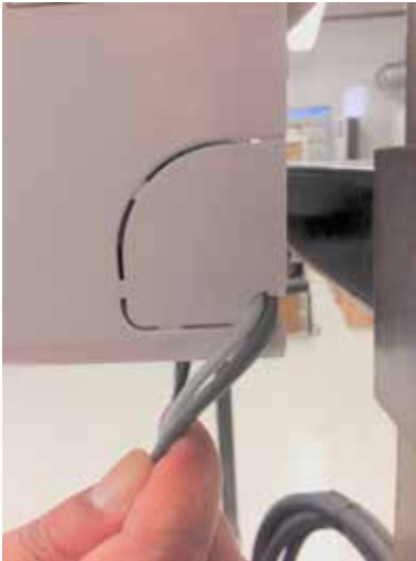
Figure 60: Indoor Unit Knockout (Communication Wires)
