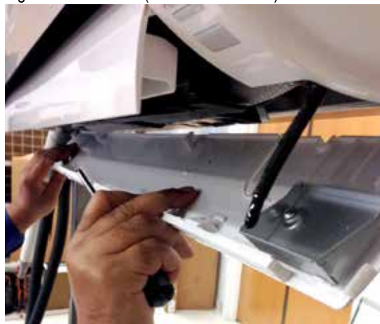
Figure 59: Remove (and Reattachment) Bottom Panel
