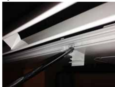
Figure 59: Remove (and Reattachment) Bottom Panel
