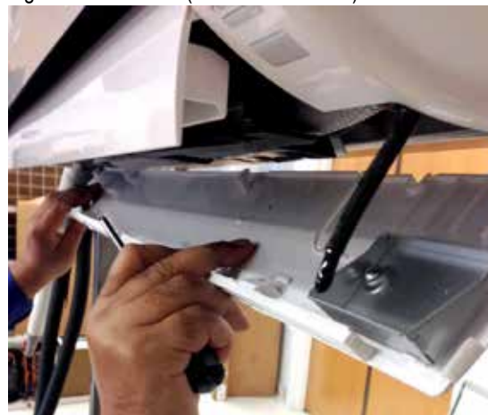
Figure 59: Remove (and Reattachment) Bottom Panel
