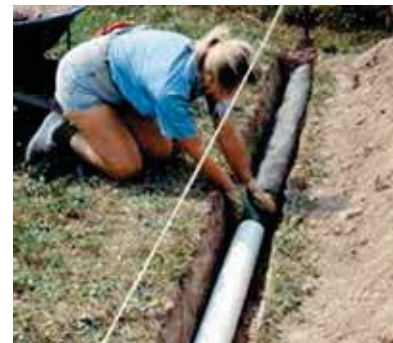
Figure 65: Underground Refrigerant Piping.
