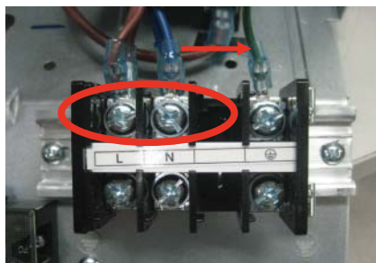
< Input Power Source Check Point >
