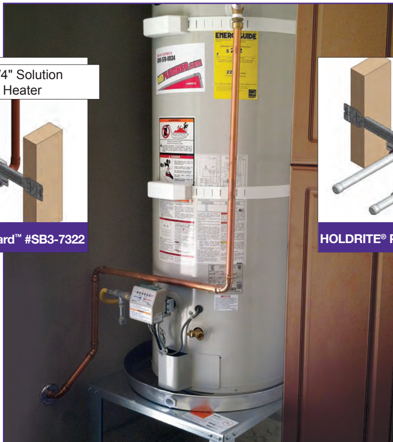
CPVC 3/4" Solution Water Heater
