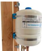
Expansion Tanks can be secured using one or two UNC1 Kits
