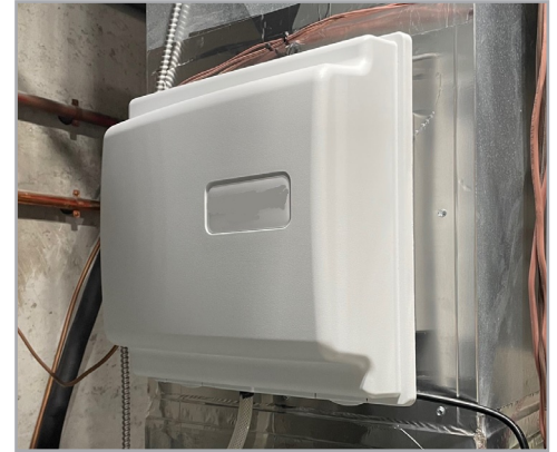
Vertical Supply Plenum Installation
