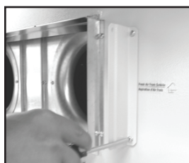
Figure 1 Support "B" installé
