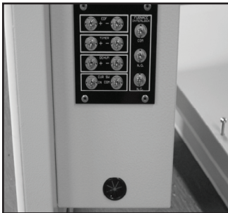
Figure 6 Insert damper motor wires through bushing
