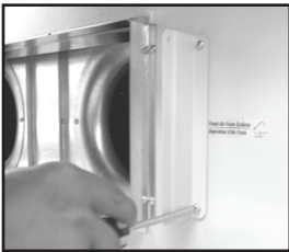
Figure 1 Bracket "B" Installed
