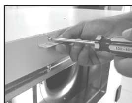
Figure 2 Support "A" installé
