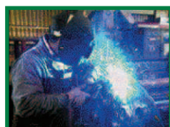
All welds completed prior to PermaGlas Ultra Coat.
