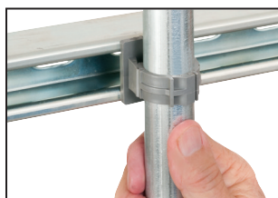
5 Secure installation of conduit to strut.
