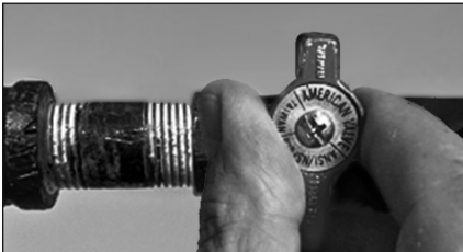
Figure 46 - Gas valve in “off” position.
