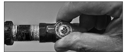
Figure 50 - Gas valve in “on” position.
