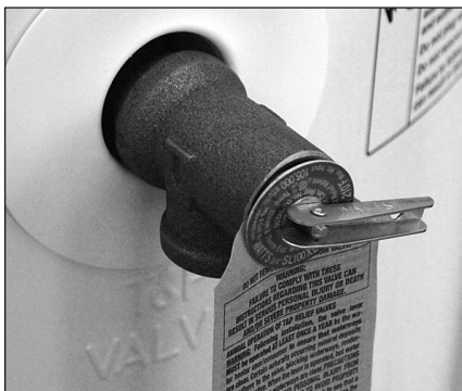
Figure 25 - Temperature and Pressure Relief Valve
