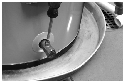
Figure 20 - Draining the old water heater.
