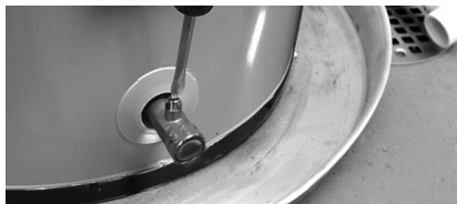
Figure 40 - Draining the water heater.
