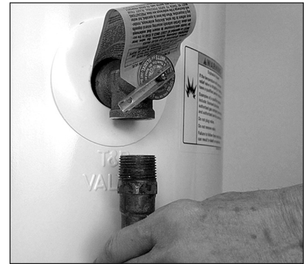
Figure 21 - Removing the T&P Relief Valve discharge pipe.
