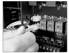
Feed wiring through hole near the top of the transformer and insert transformer plug into the socket.
