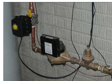
Common TickerValve Installation
