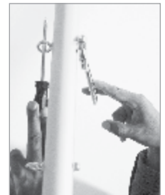
Figure 9: Use two fingers to tighten bolts
