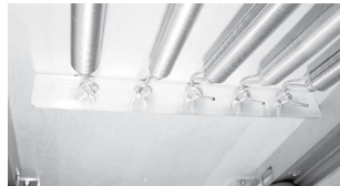
Figure 3: Springs hooked downward
