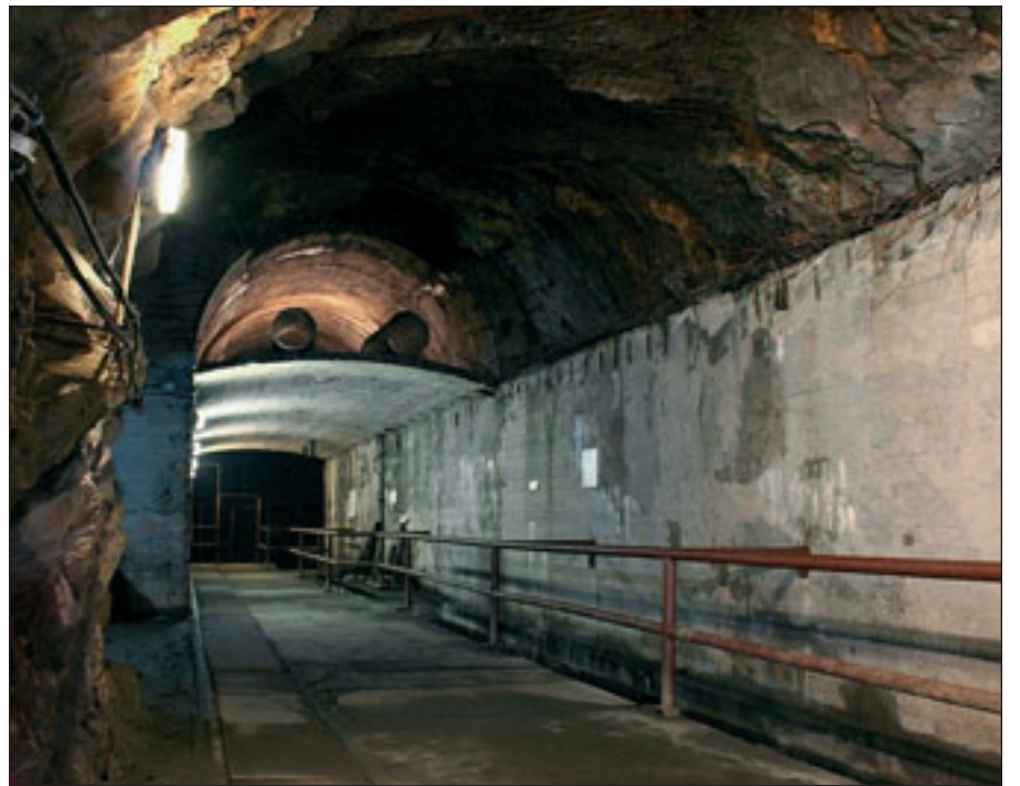
Tunnels in the Owl Mountains, Project Riese
