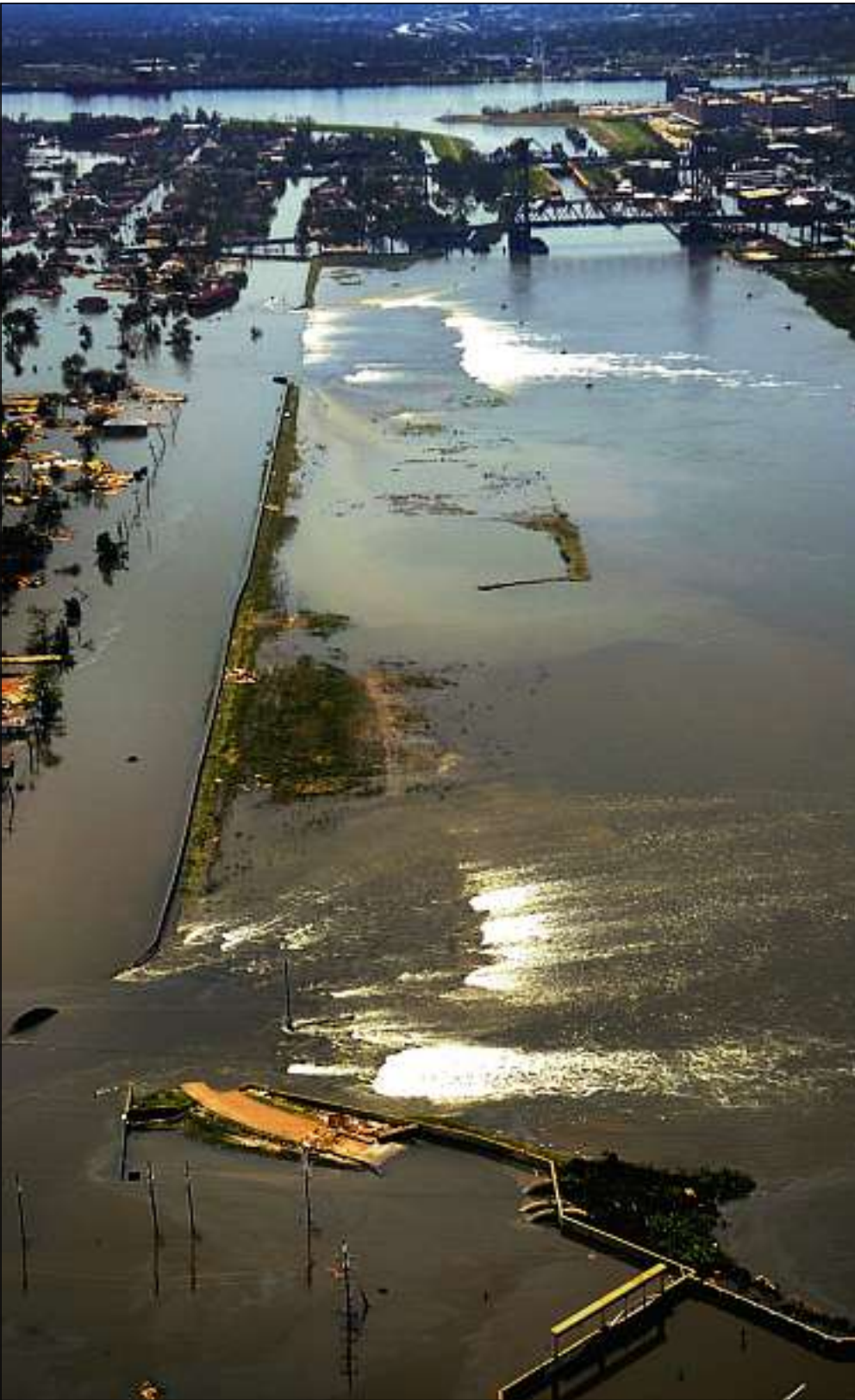
Hurricane Katrina caused the two levee breaches shown Tuesday. Failure of the levee system resulting from the storm left much of New Orleans under water.
