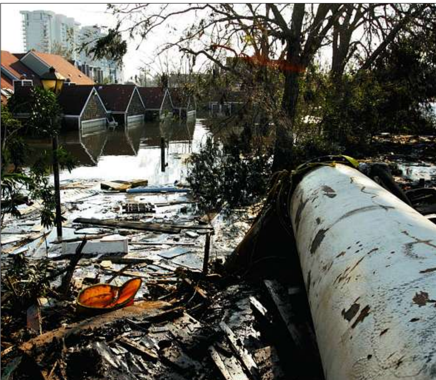
Water is pumped out of a flooded Metairie, La., subdivision today through a 30-inch pipe that sucks out 27,000 gallons of water per minute. Engineers have managed to plug a major levee break.
