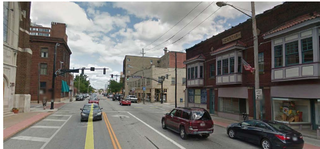
Context: Detroit Avenue Looking West with Curtis Block
