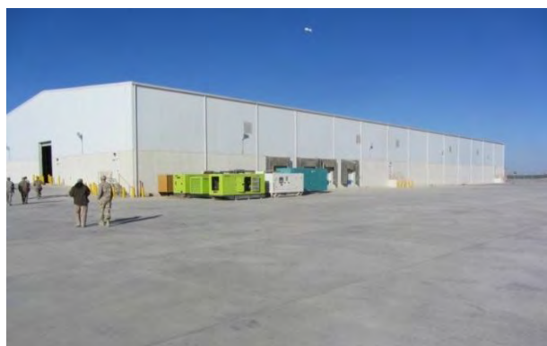
Photo 1 - Warehouse Building at KAF
