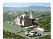
中国实验快堆核岛自动消防系统总包完成 Sureland was the total solution provider for the automatic fire extinguishing system for CERF of China Institute of Atomic Energy
