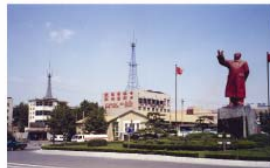
武汉钢铁集团，曾安建楼近十多年，总承包实施多个重要消防项目并成功扑救1997年“4.28”火灾 Wuhan Iron and Steel Group: Sureland has provided total fire protection solutions for more than ten years and implemented many important fire protection projects and successfully put out the “4.28” fire disaster
