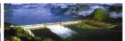
晋安为长江三峡电站、大坝及永久船闸自动报警系统、网络监控系统、专用报警系统工程均由晋安总包完成 Sureland was the total solution provider for the automatic fire extinguishing system for “Three Gorges” Project
