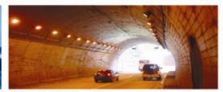
晋安为、超高压输电线路自动消防系统 Fire Protection Systems for Yuxuan Highway and Kunshi Highway
