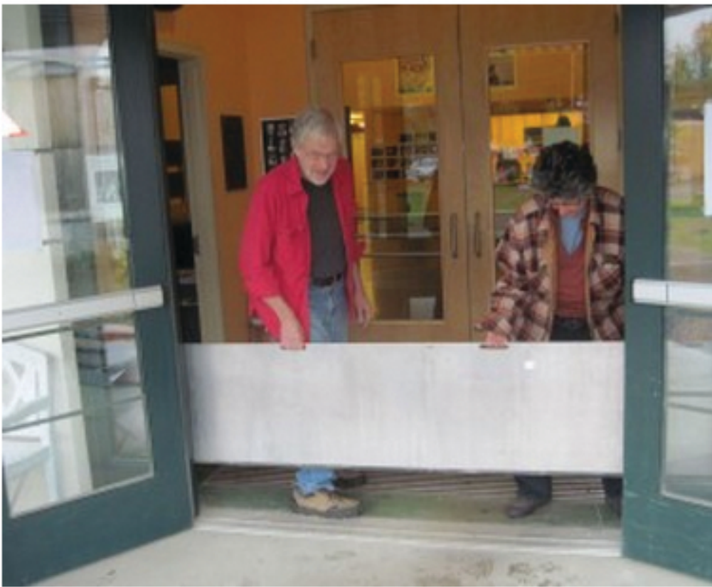
The shields were easily inserted in the channels to provide a watertight barrier.
